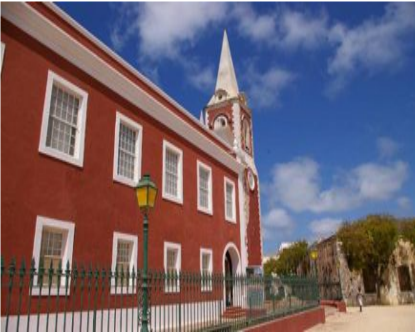
Rehabilitated building on Ilha de Mozambique
